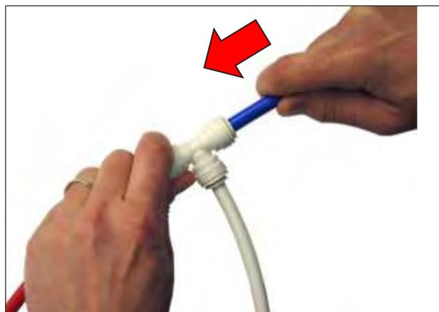
4. Pull on the fitting to check that the connection is secure. Test the system for leaks prior to leaving the site. (Fig. 4)
